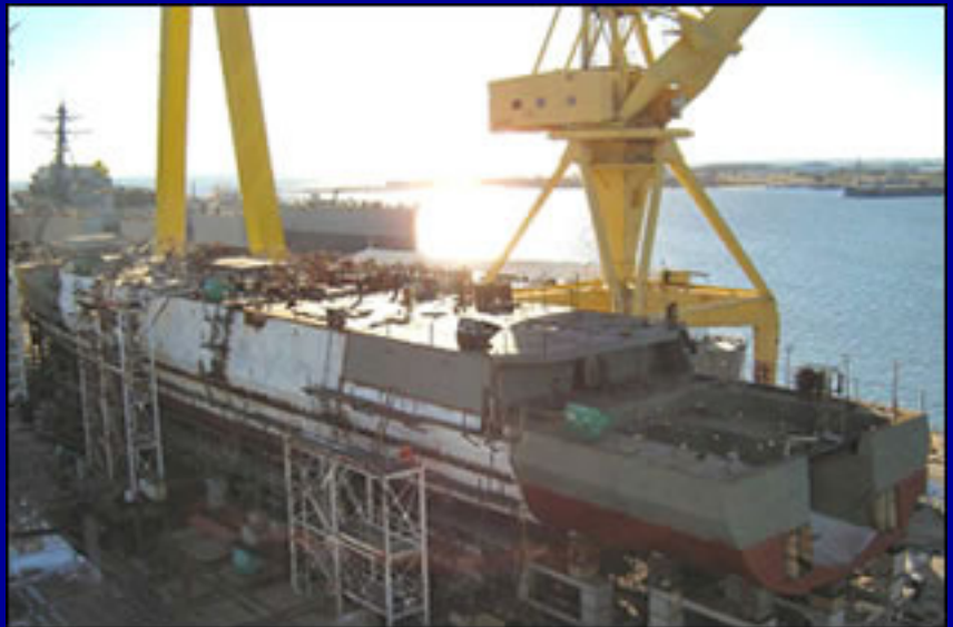
The first National Security Cutter. The aft end of the extended flight deck and the stern ramp/boat stowage area are featured above. (Photo courtesy of Northrop Grumman)
